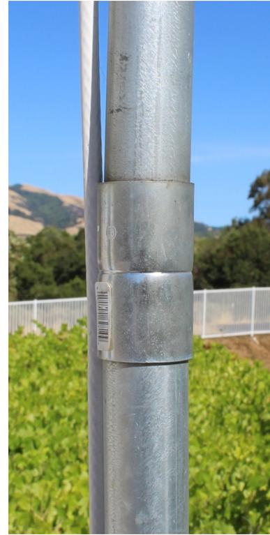
10' 1" Conduit Pipe and 5' Pipe Engaged by Coupling
