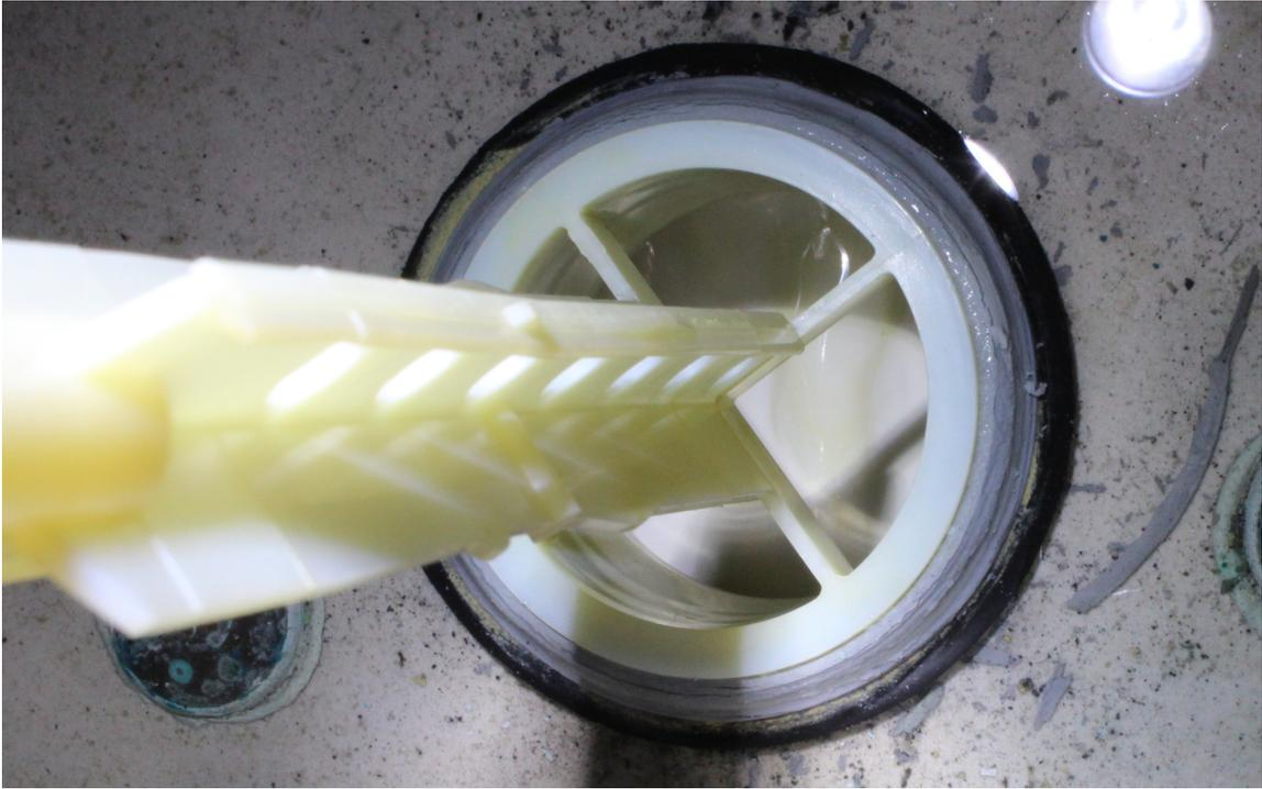
Black Deteriorated Flush Valve Gasket Leaking Tank Water to Toilet Bowl All the Time
