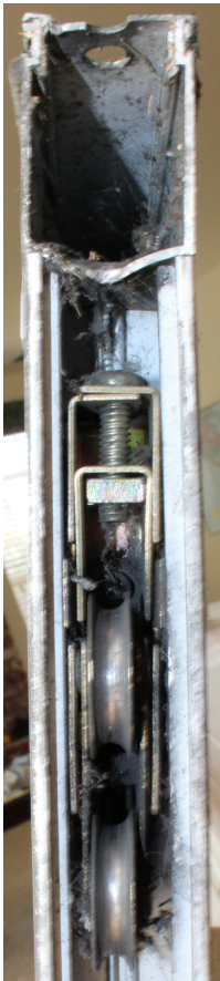
Wheel roller assembly (LH) Wheel roller assembly (RH)
