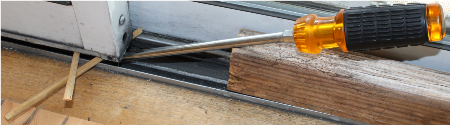
From left; Chop sticks for keeping door bottom up, Long flat driver working as a leverage to make the right-hand side door bottom up, 2x2 lumber for leverage platform
