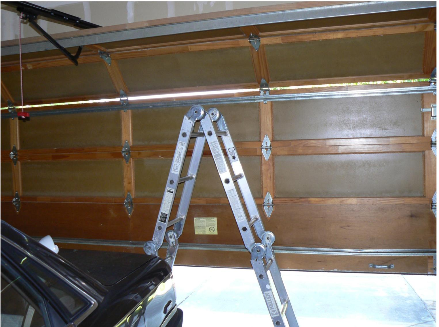
Garage door keeps opening steadily balancing heavy door weight (downward) & hoist energy (upward) generated by torsion spring. Garage door opener (Electric motor) generates smaller power to SHIFT the door up and down.
