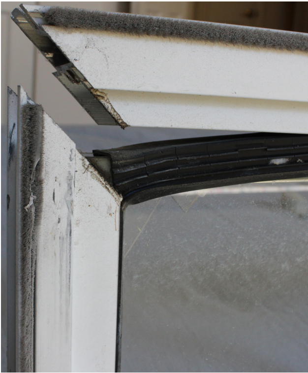
Frames separated after unscrewed
