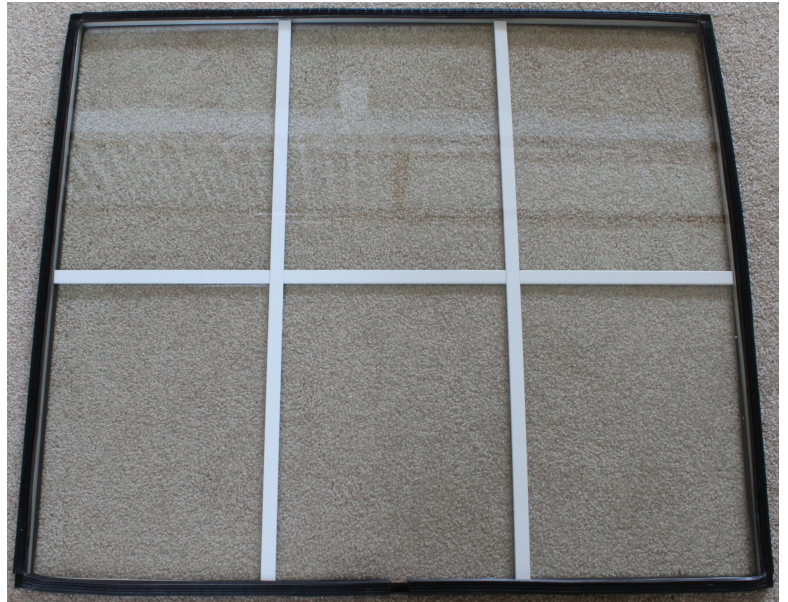
Gasket attached to glass
