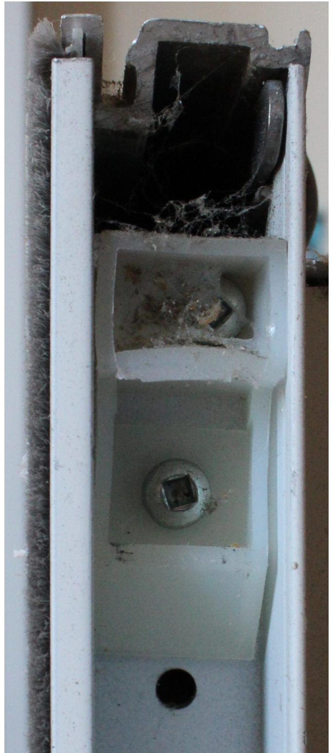
Four square head (Robertson) screws attach four window frames together at four corners
