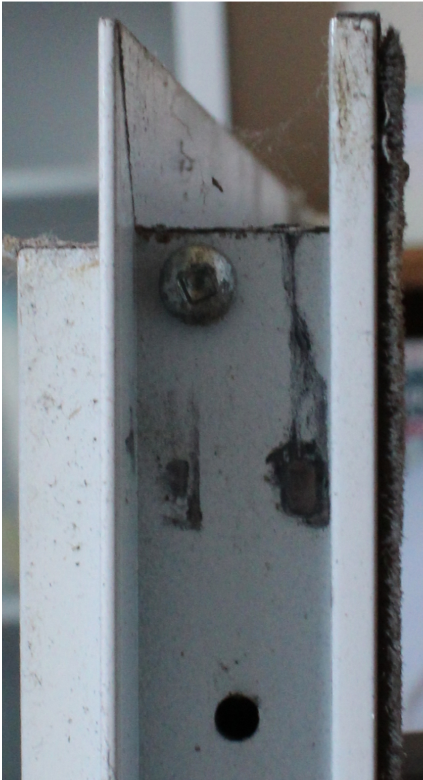
Four square head (Robertson) screws attach four window frames together at four corners
