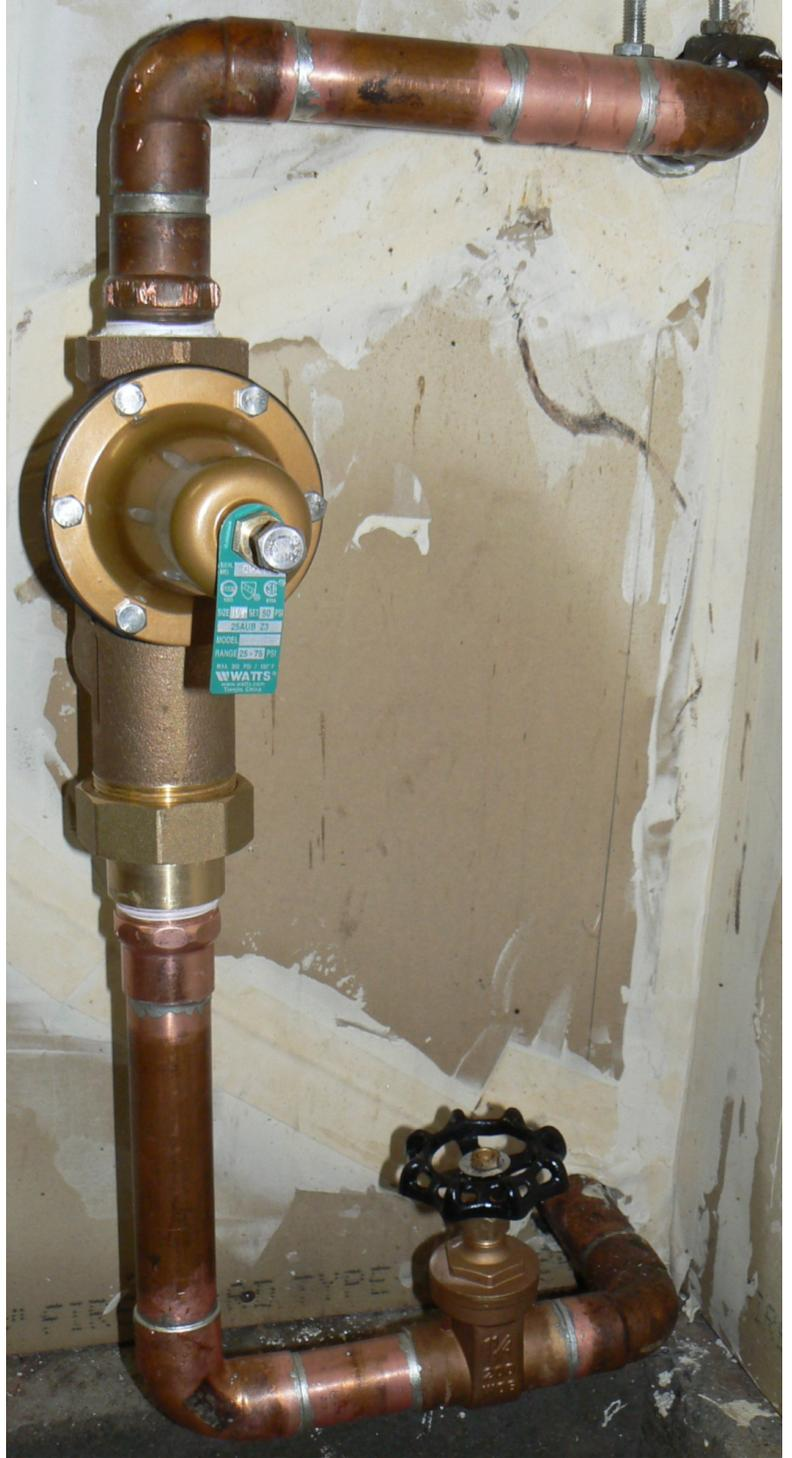
Replaced (1 1/4" Copper Pipe and Valves)
