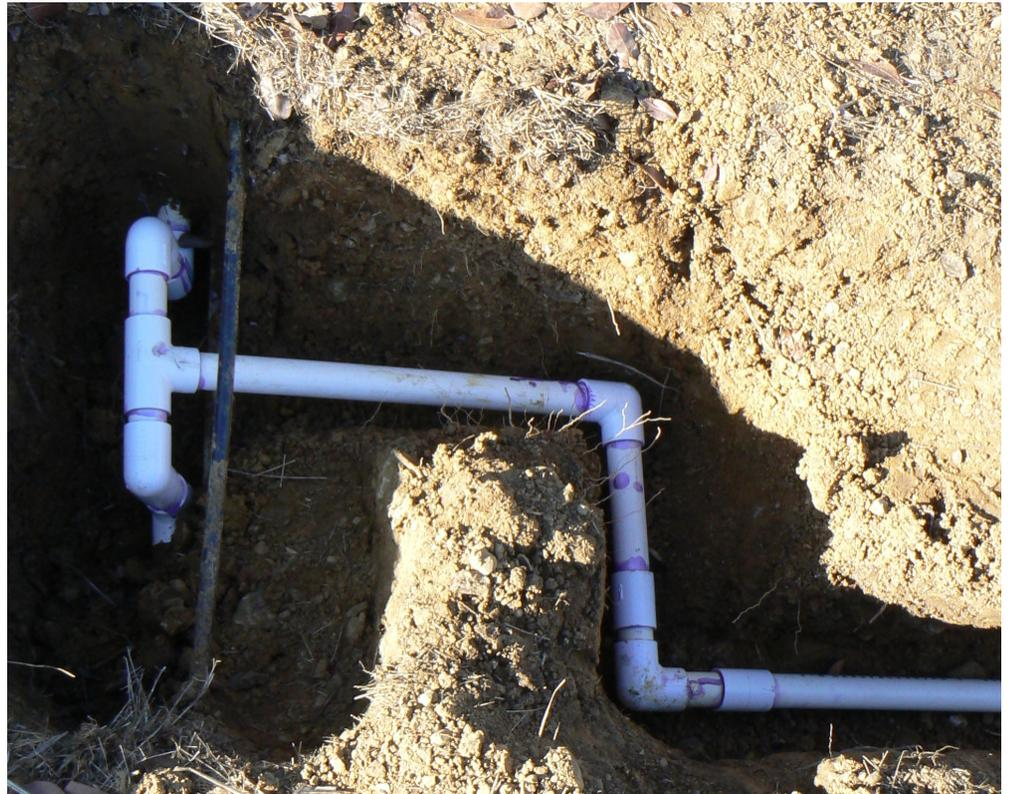
1" PVC piping for water drip line at sloping ground needs a certain special pipe fitting technique.
