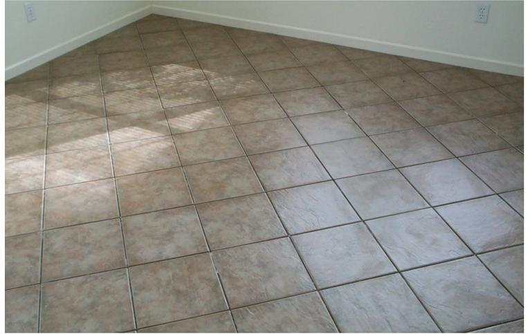
Tiles Glued to Floor by Tile Adhesive (Before Grout)
