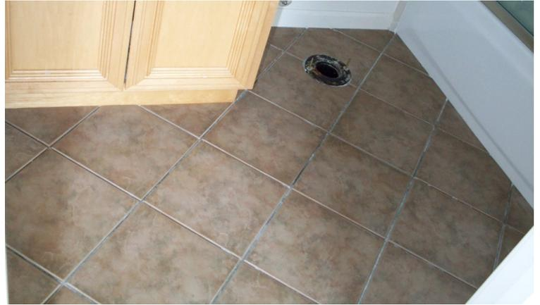
Tiles Glued to Floor by Tile Adhesive (Before Grout)
