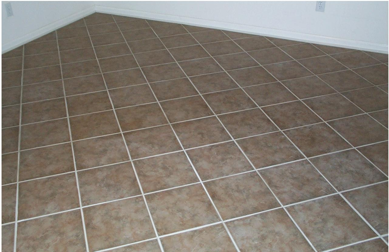
Tiling Done (After Grout & Grout Seal)
