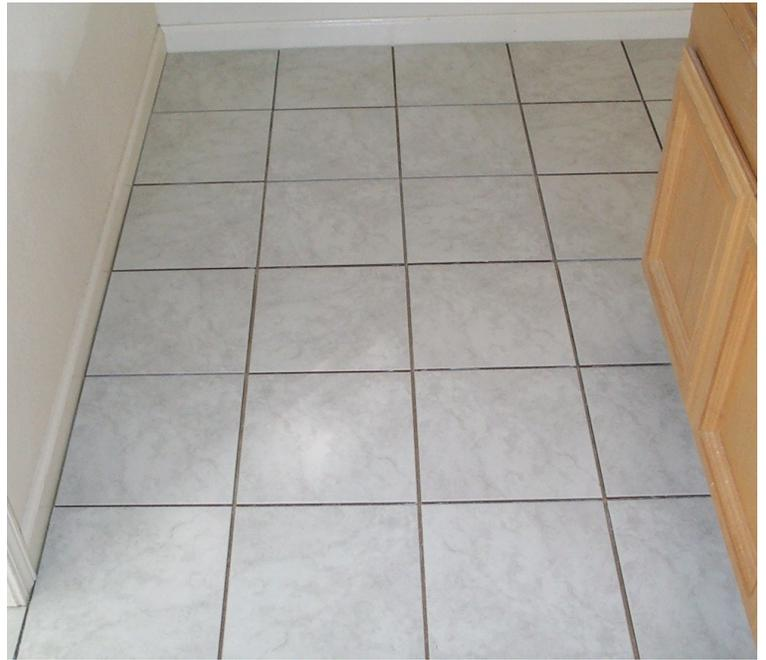
Tiles Glued to Floor by Tile Adhesive (Before Grout)
