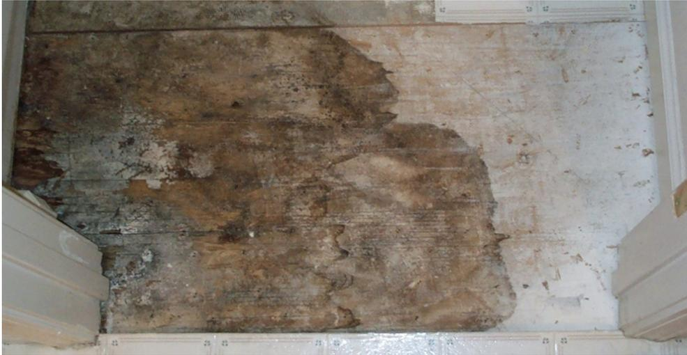
Water Leak Found after Removing Vinyl Flooring
