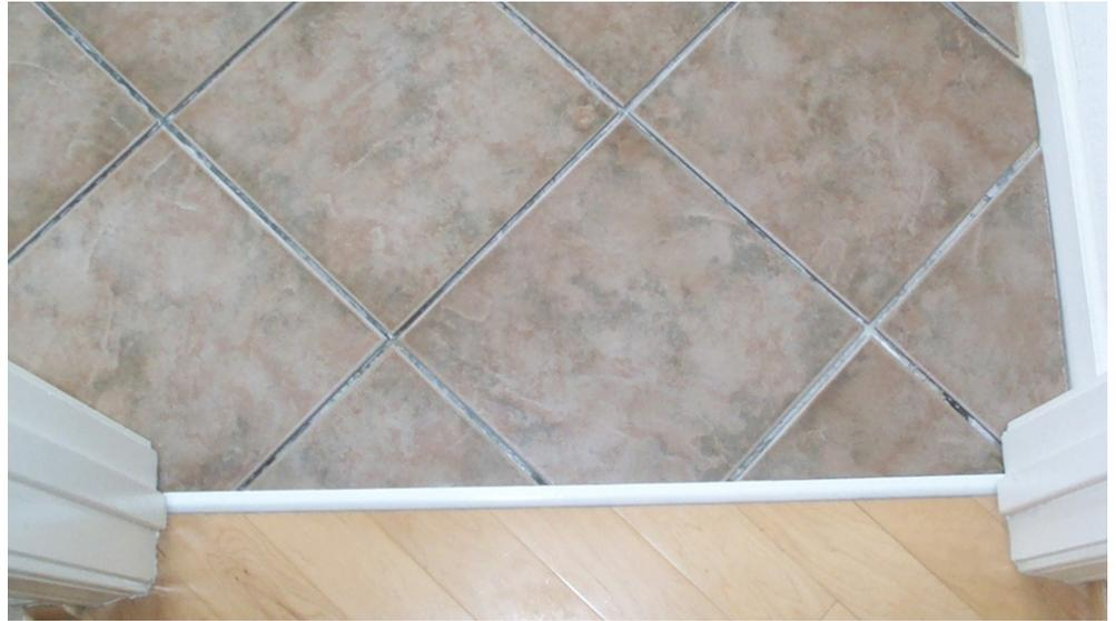
Tiles Glued to Floor by Tile Adhesive (Before Grout)
