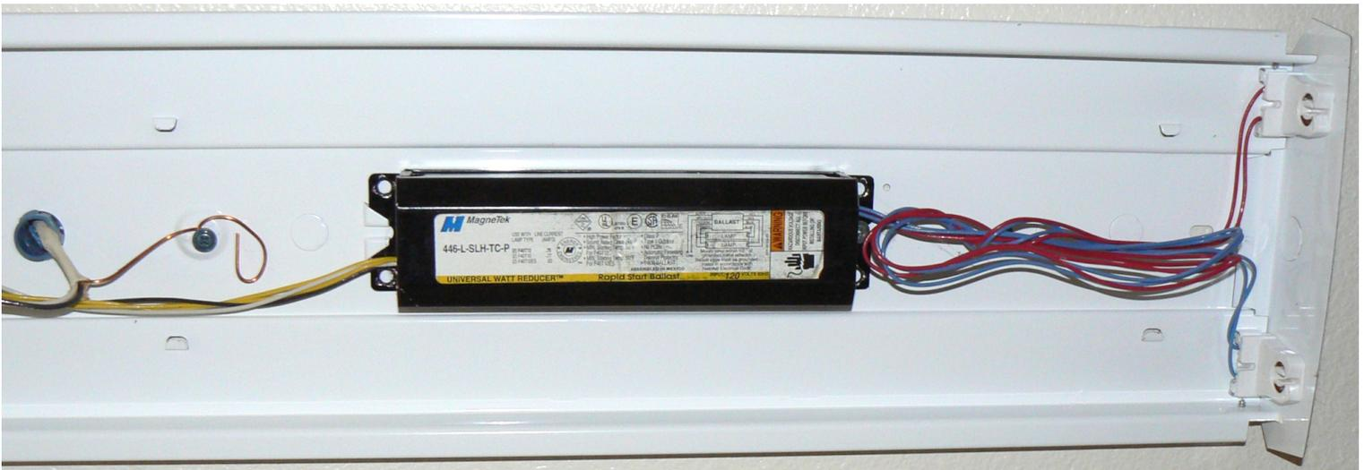
Original Wiring for Fluorescent Tube Housing (Right Portion)
