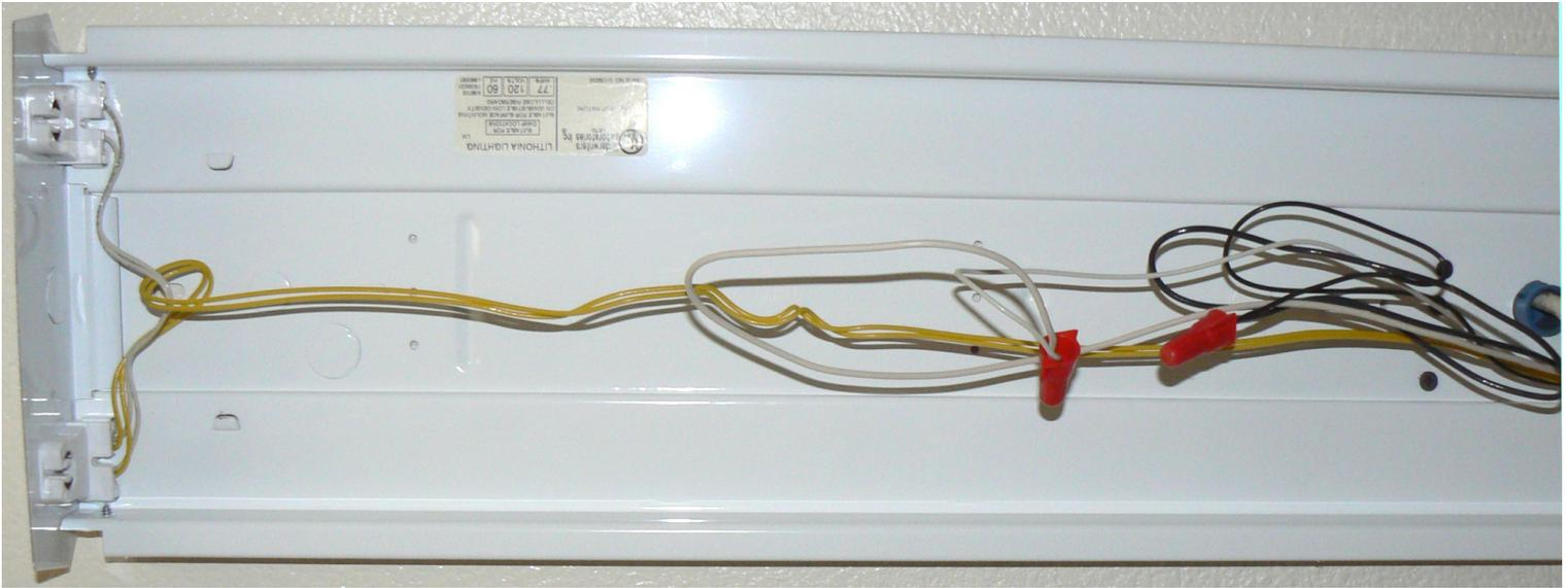
Original Wiring for Fluorescent Tube Housing (Left Portion)
