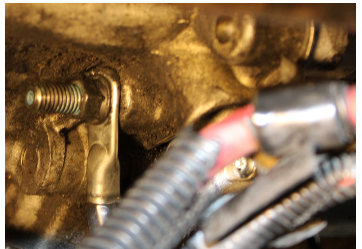
Thick ground wire (Black) directly from battery fastened by a Stud Bolt#1 and a nut
